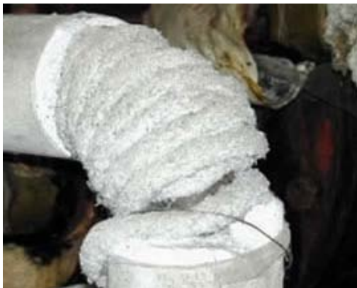
Asbestos Rope and Asbestos Insulation
